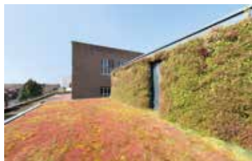
Barley Mow Centre, Chiswick: 3,000 sq. ft. of green roof and wall.
