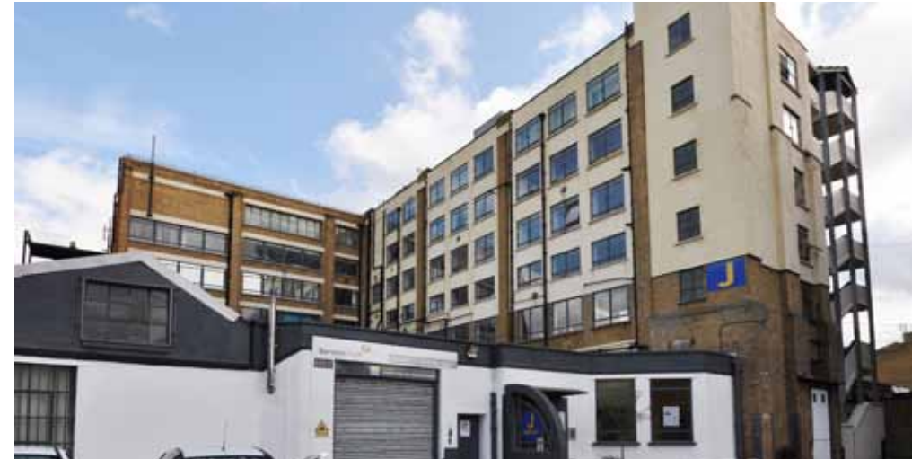
TOWER BRIDGE (BLOCK B)
