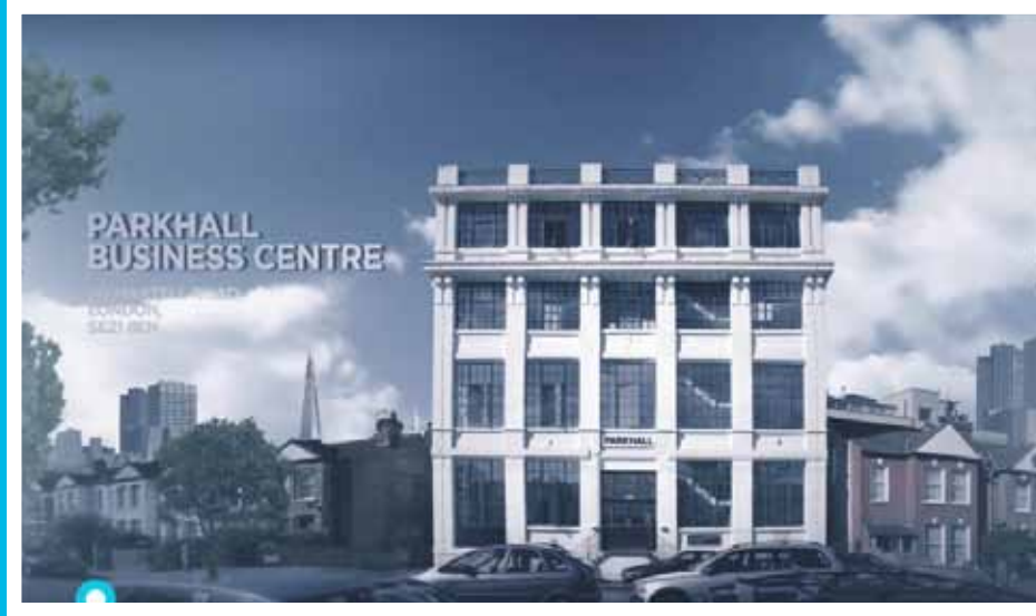
PARKHALL BUSINESS CENTRE REPOSITIONING
