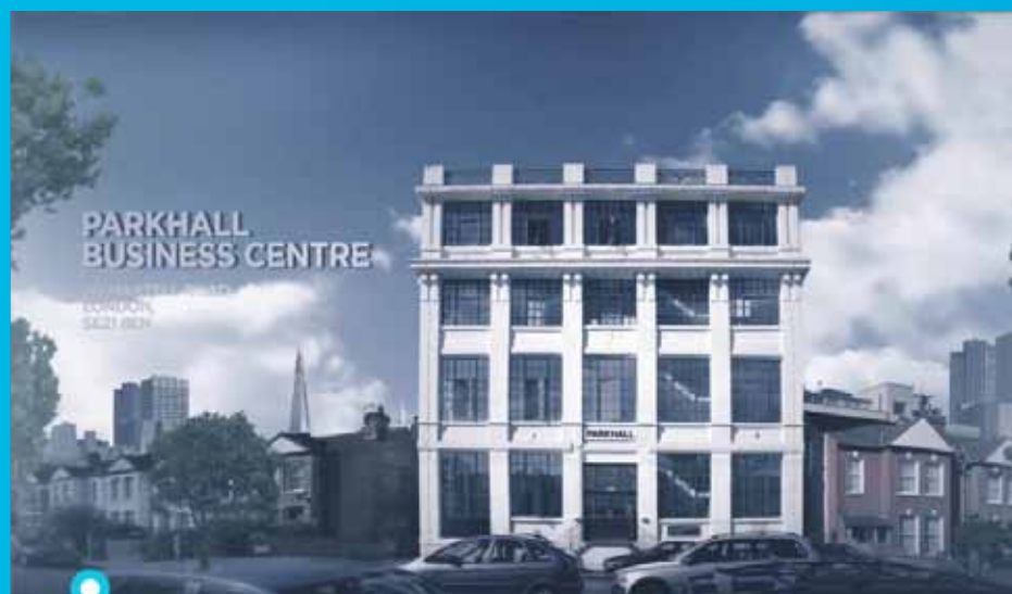
PARKHALL BUSINESS CENTRE REPOSITIONING
