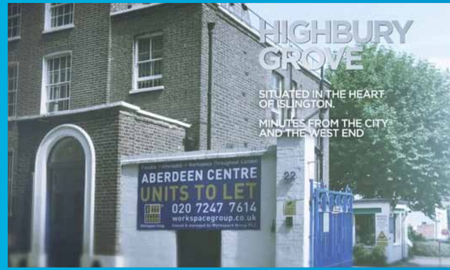
HIGHBURY GROVE REDEVELOPING
