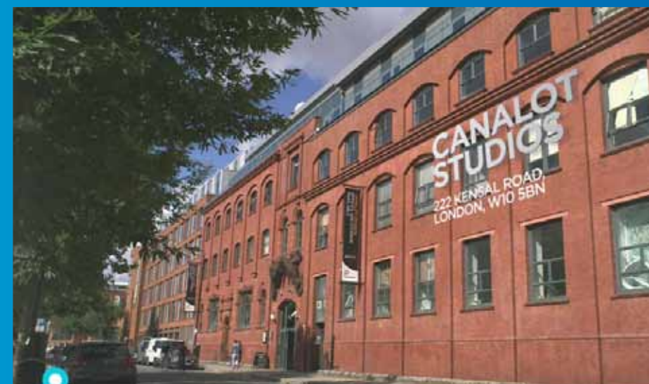
CANALOT STUDIOS REFURBISHING
